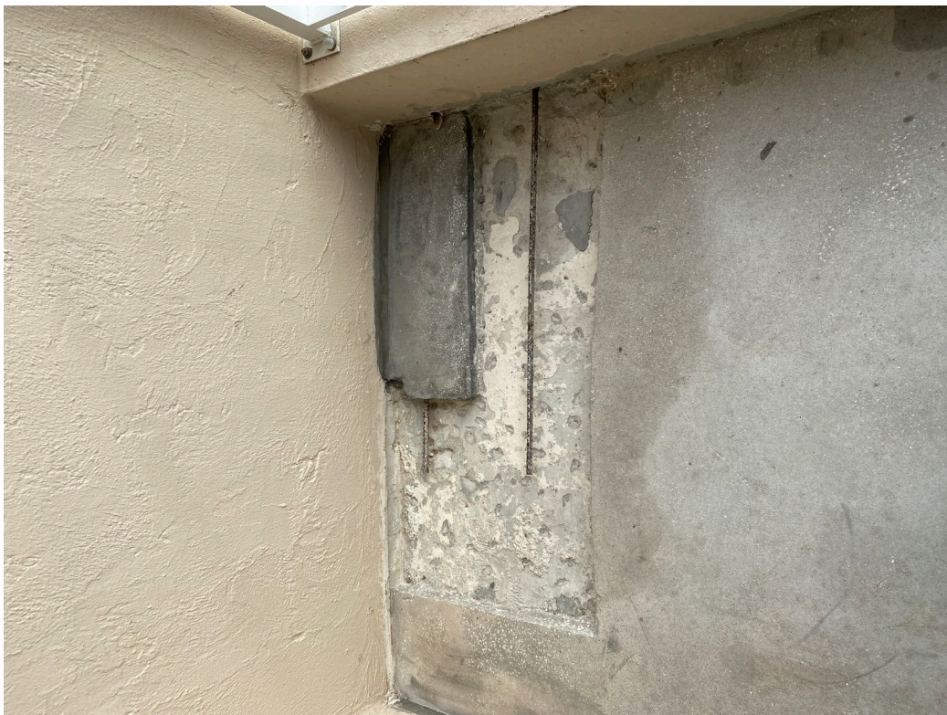
Picture 2: Typical topping repair
