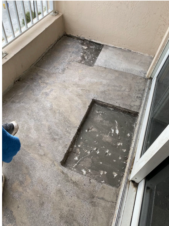
Picture 1: Typical topping repair
