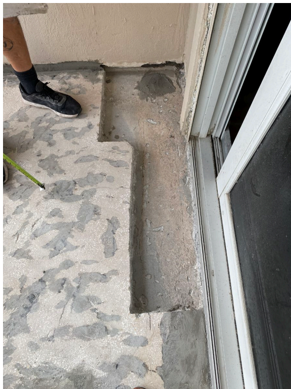
Picture 3: Cracks in the precast panel of Unit 108
